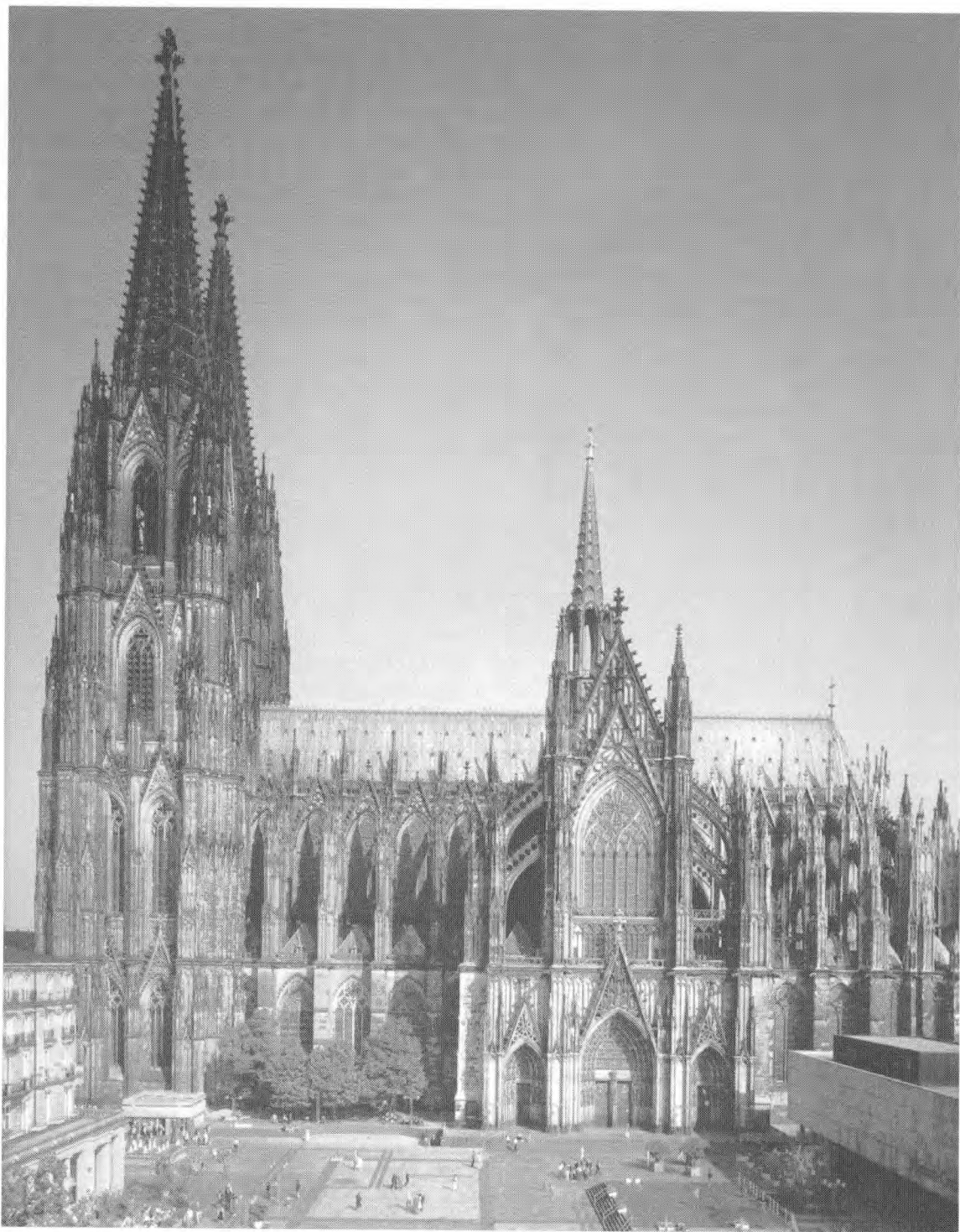
Fig. 1.54. The Cologne Cathedral as it is today. Cologne, Germany. Taken from [1017], photograph 3.
